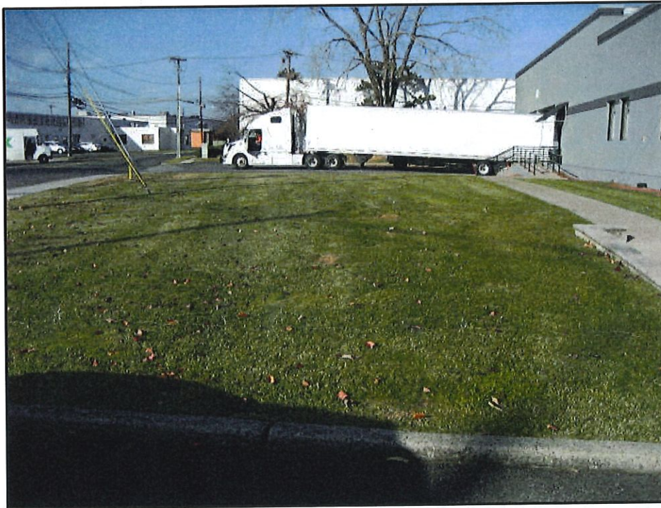
Photo 10 – Engineering Control C-4: Vegetative Cap Protective of Human Health and the Environment
