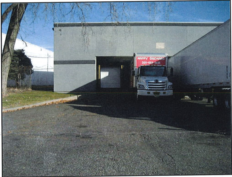
Photo 5 – Engineering Control C-2: Asphalt Cap Protective of Human Health and the Environment
