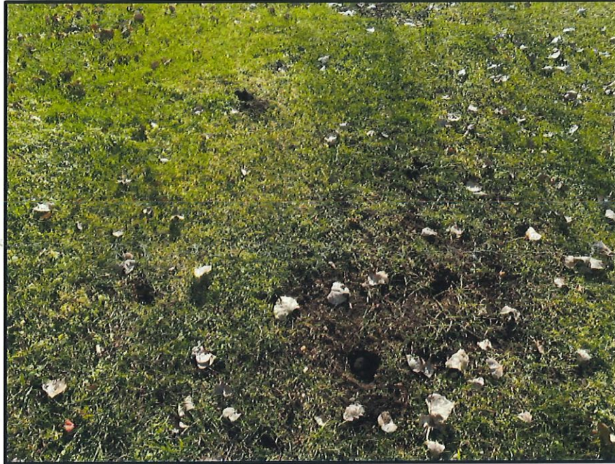
Burrow Holes Before Repairs in the Southwest Landscape Cap 11/30/2023
