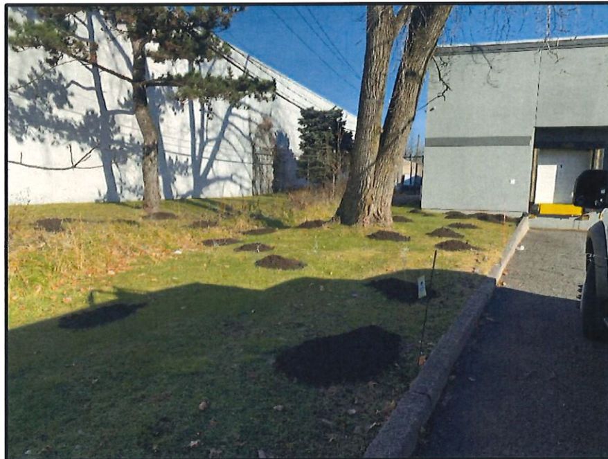
Burrow Holes After Repairs in the Southwest Landscape Cap 12/18/2023
