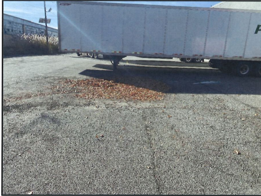
Before Repairs Northeast Asphalt Cap 11/30/2023
