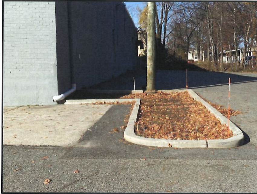
Before Repairs Northeast Landscape Cap 11/30/2023
