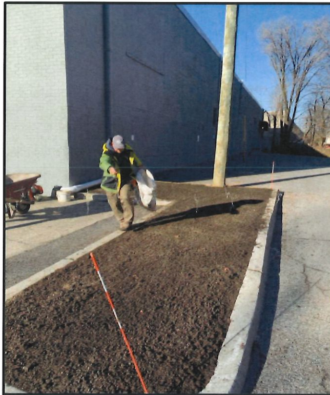
After Repairs Northeast Landscape Cap 12/18/2023
