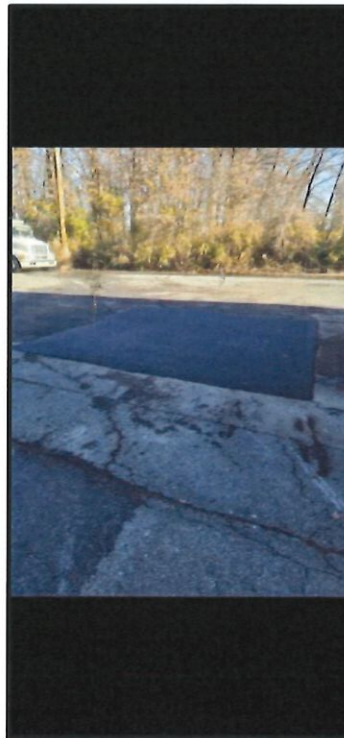
After Repairs Northeast Asphalt Cap 12/18/2023
