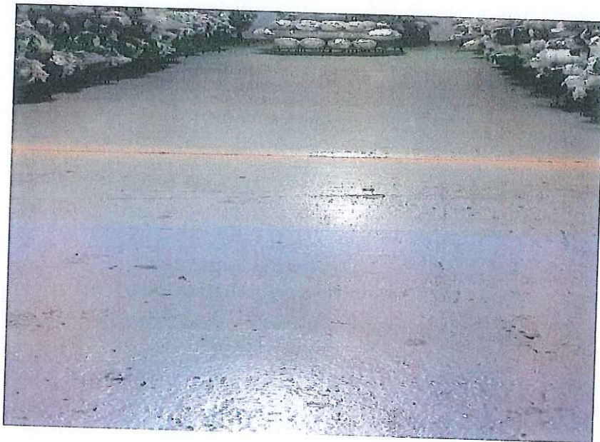
Photograph #15 – View of the concrete cap of the subject property.
