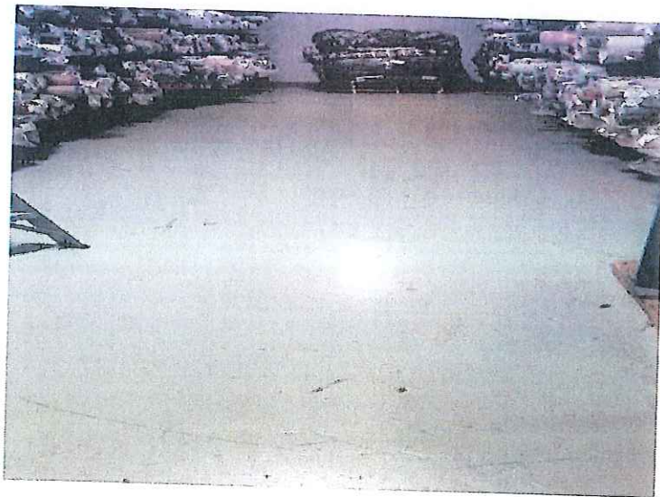
Photograph #18 – View of the concrete cap of the subject property.
