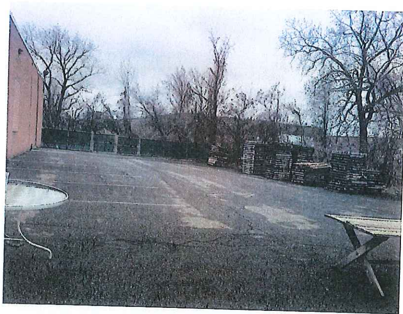
Photograph #10 – View of the asphalt cap of the subject property.
