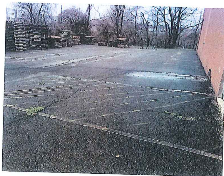
Photograph #12 – View of the asphalt cap of the subject property.
