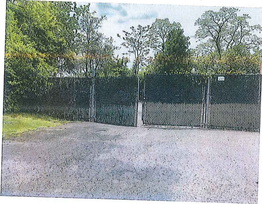
Photograph #9 – View of the asphalt cap and fence of the subject property.
