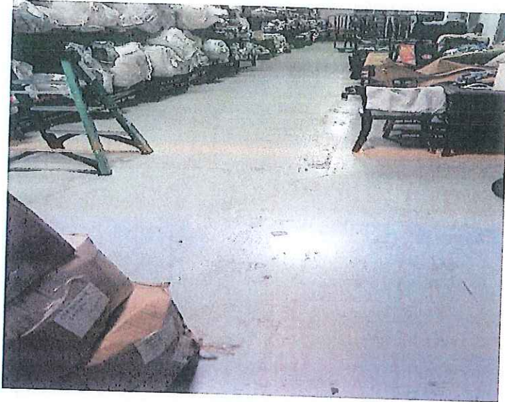
Photograph #17 – View of the concrete cap of the subject property.
