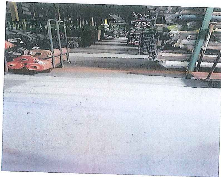
Photograph #19 – View of the concrete cap of the subject property.
