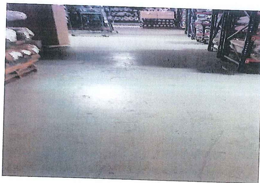
Photograph #16 – View of the concrete cap of the subject property.
