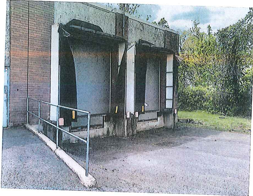
Photograph #13 – View of the asphalt cap of the subject property.
