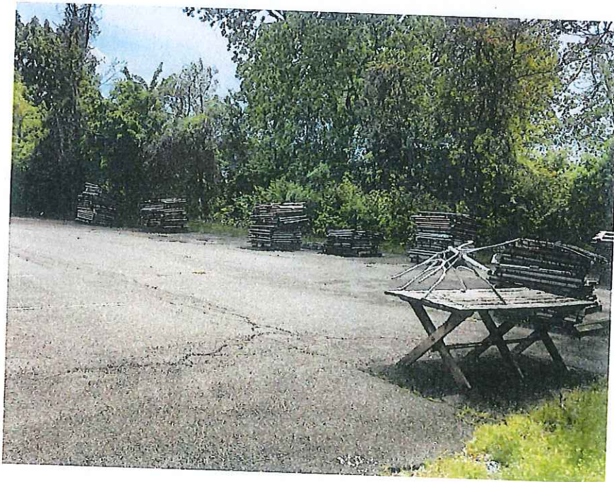
Photograph #16 – View of the asphalt cap of the subject property.
